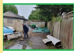
The plan for the next few months is to replace the old asbestos roof and guttering, repair the brickwork and fit some new doors. Some of the plumbing also needs renewing, a new fence added and a concrete slab laid where the soil and rubble were removed. We then hope to repaint both outside and inside to tidy it up and get it ready for the winter months. This should give us a refreshed storage site that will last for many years to come.
